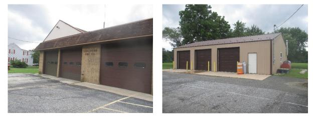
Stormwater currently drains from the property and the roofs of the buildings without downspouts. A cistern, as well as a downspout, can be installed on the northwest corner of the west building to capture stormwater runoff. The water can then be used for washing vehicles or for other non-potable uses such as car wash fundraisers or watering existing landscape plants. A preliminary soil assessment suggests that the soils have suitable drainage characteristics for green infrastructure.
