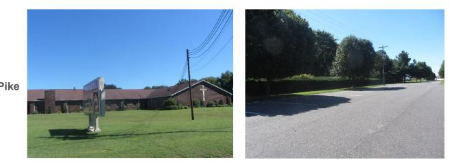
Stormwater is currently directed to existing catch basins throughout the parking lot. Parking spots on the far east and west sides of the parking lot can be replaced with porous asphalt to capture and infiltrate stormwater. A preliminary soil assessment suggests that the soils have suitable drainage characteristics for green infrastructure.
